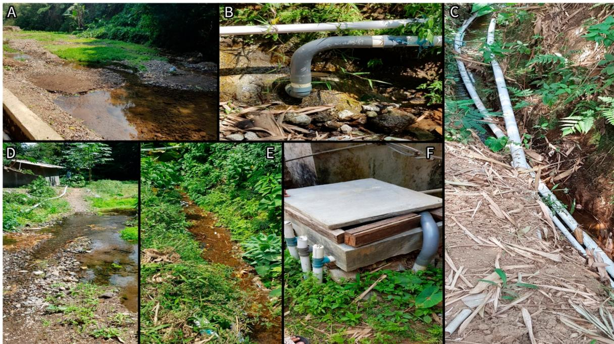
**Figure 3.** Flow of water in Losari. (A,D,E)—Neighboring environment of groundwater spring. (B,C)—Pipes from spring to holding tank. (F)—Water holding tank.
