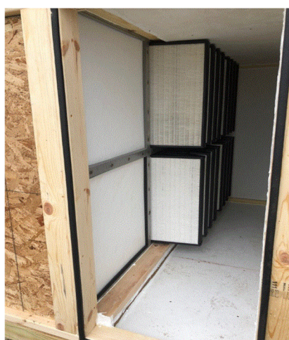
Figure A.5. Picture of the inside of the MERV filtration unit.
