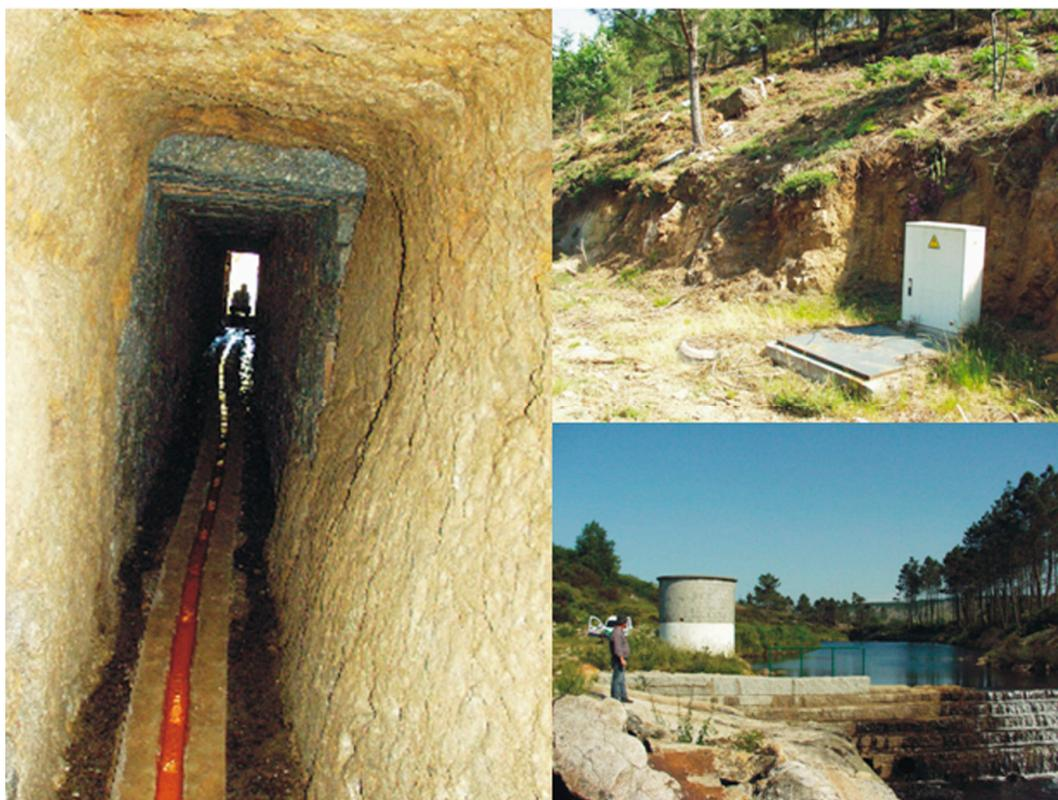
**Figure 3.** Sources of groundwater used in Vila Pouca de Aguiar for public supply of drinking water: left panel—spring/gallery; upper right panel—drilled well; lower right panel—alluvial well.
