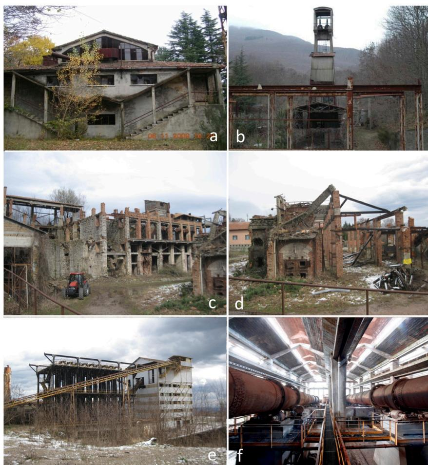
**Figure 4.** Buildings and mining structures analyzed in this work: (a) miners' dressing building; (b) Garibaldi well; (c) old driers and condensers; (d) old mud deposit and furnaces; (e) Nesa furnace and condensers; (f) building hosting the Gould furnaces.
