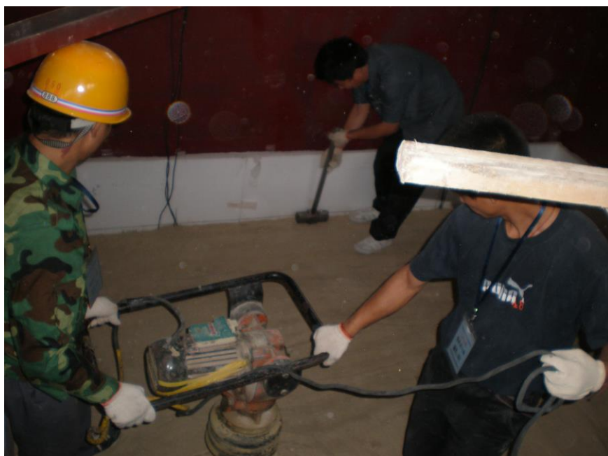
Figure 7. Artificial consolidation and mechanical compaction.
