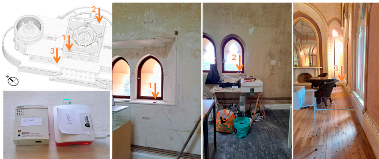
Figure 4. Equipment position in the palace, in situ survey from 8 April to 16 July 2024, OMRON and HOBO; positions 1 and 2 are on windowsills on the second floor (southwest and northeast workroom), and position 3 is in a wood floor corner on the ground floor (dining room).
