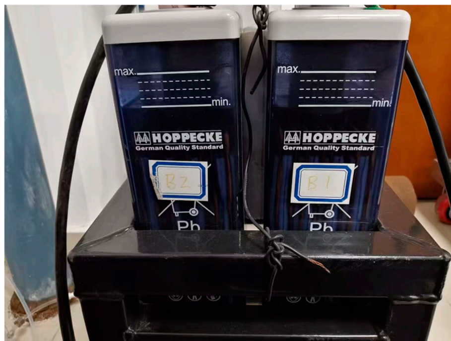
Figure 1. Upper and lower limit markings for the liquid level of lead-acid batteries.
