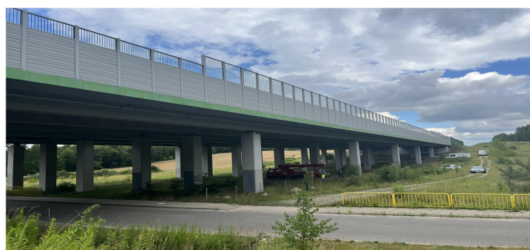
Figure 1. General view of the viaduct in Plichtow [35].
