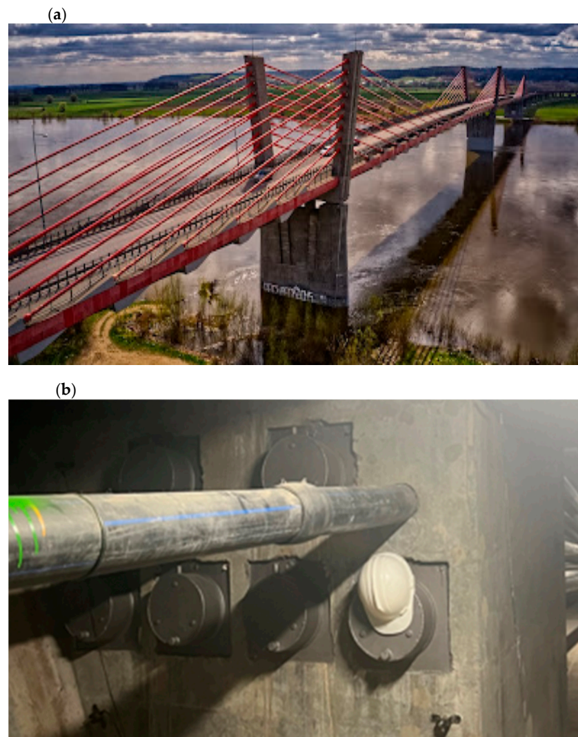
Figure 1. View of the bridge (a) with an internal anchor block for prestressing cables (b).
