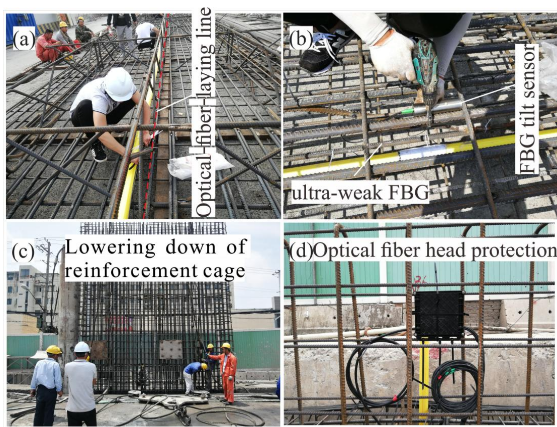
Figure 12. Field installation of optical fiber sensor: (a) optical-fiber-laying line; (b) installation of ultra-weak FBG and FBG tilt sensor; (c) lowering down of reinforcement cage; (d) optical fiber head protection.
