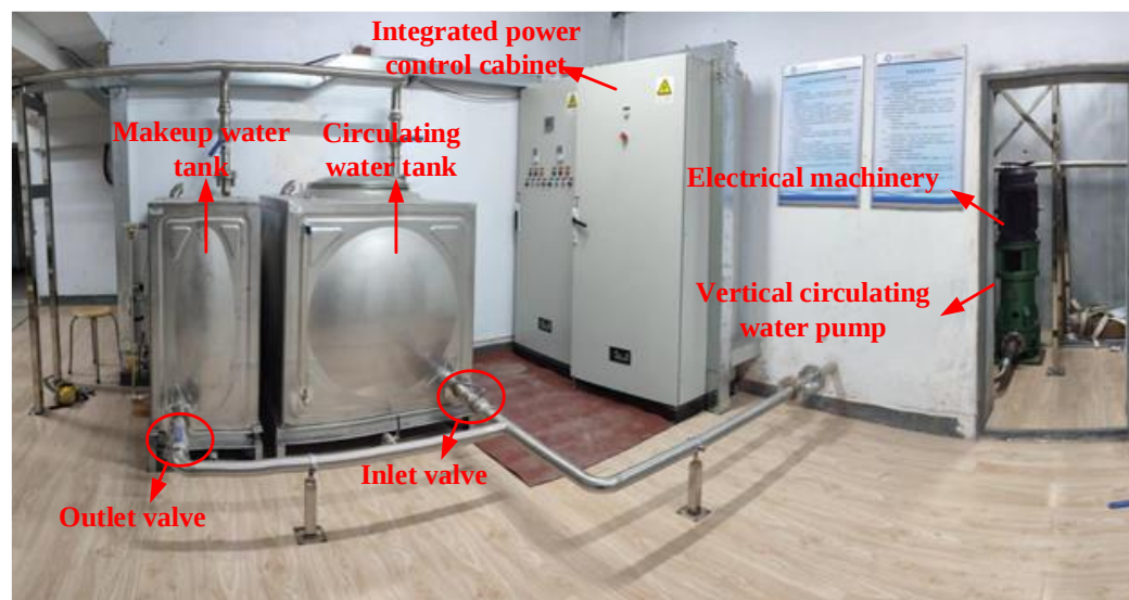
Figure 4. Actual effect diagram of the experimental bench for the rolling bearing failure of a circulating water pump.
