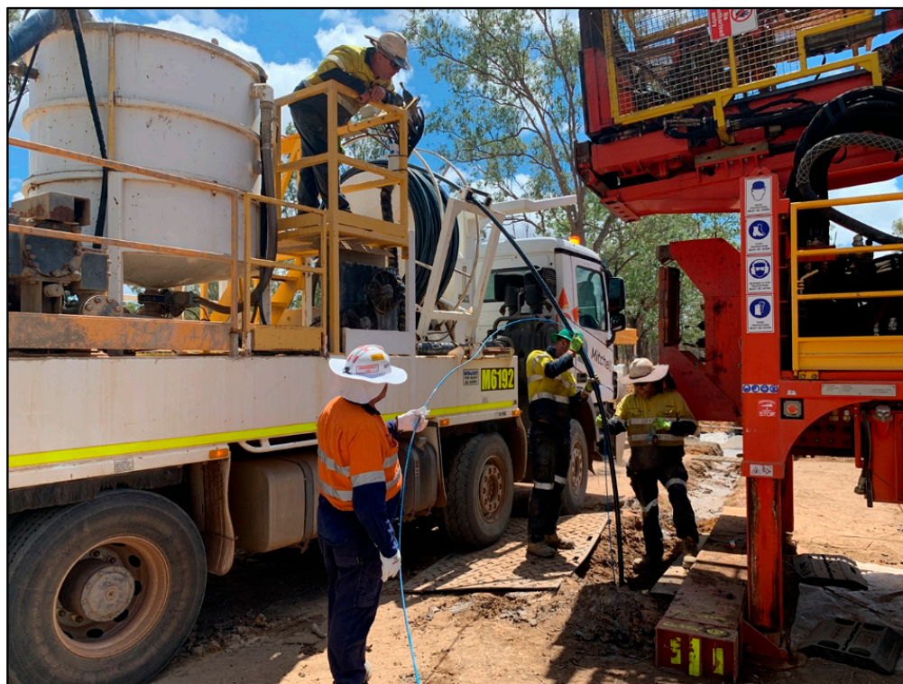
Figure 2. Installation of the fibre optic cable on a poly pipe to Borehole 2. The polyethylene pipe is attached to a grouting truck that was used to cement the borehole through the pipe.
