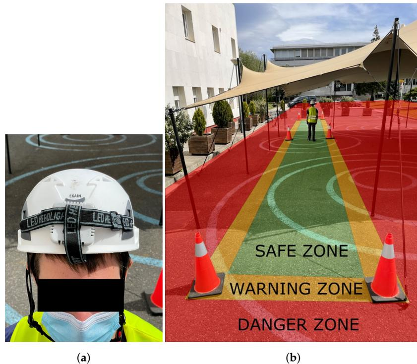
**Figure 2.** (a) Tag on hard hat of worker and (b) deployment of safety system with marked zones.
