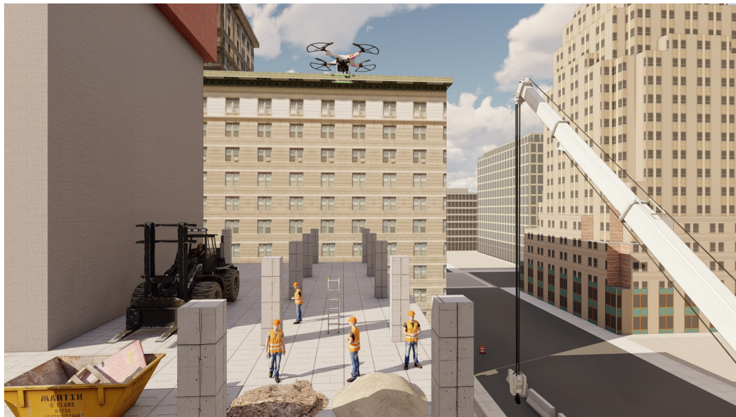
Figure 3. Layout of the Construction Site Monitoring Using UAV.
