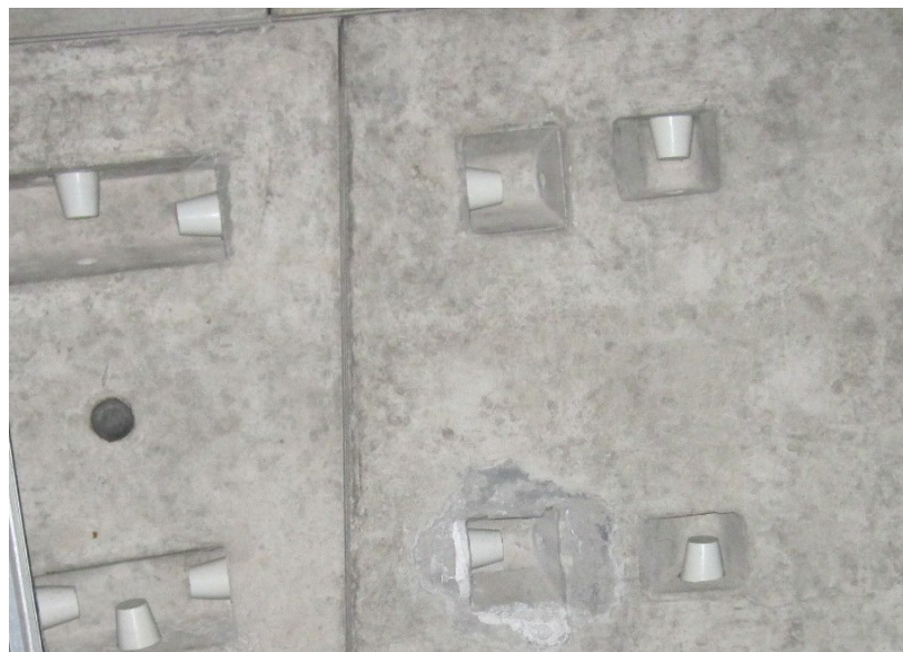
Figure 9. Images of the underground structure without water leakage.
