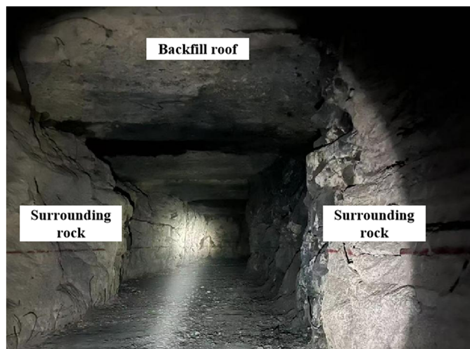
Figure 1. Field engineering structure about backfill–rock.
