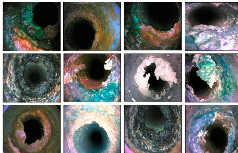
Figure 7. Grease blockage frames in the S-BIRD dataset.
