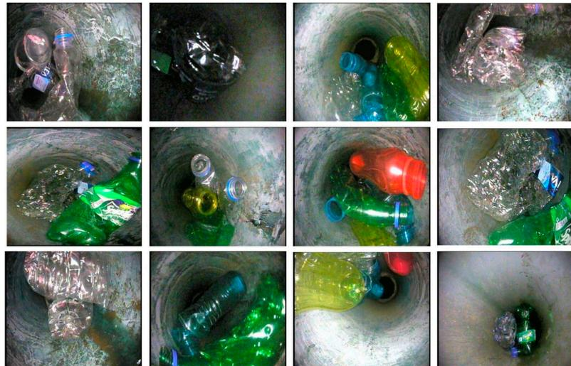
Figure 6. Plastic blockage frames in the S-BIRD dataset.
