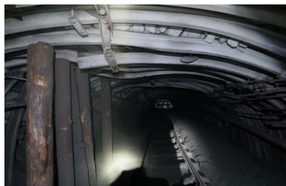
Figure 2. Temporary supports from wooden posts.
