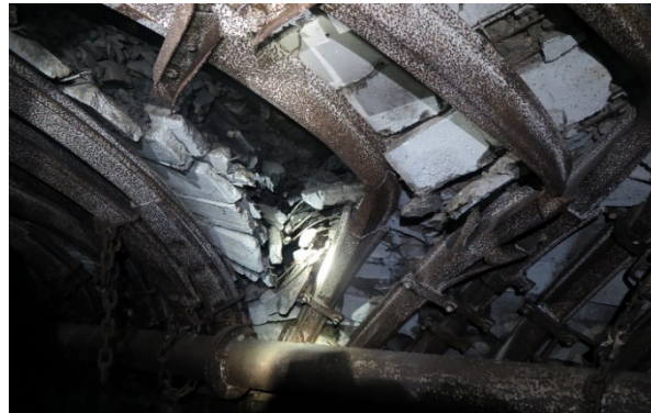
Figure 1. The destruction of the mine support under the change of rock pressure.
