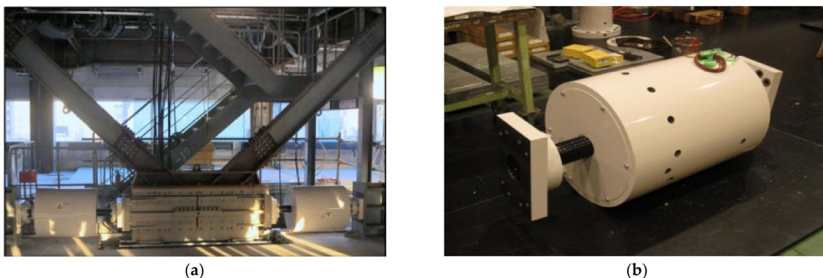
**Figure 6.** (a) Tuned viscous mass damper coupled to a chevron bracing equipping a building in Sendai, Japan; (b) tuned viscous mass damper device.
