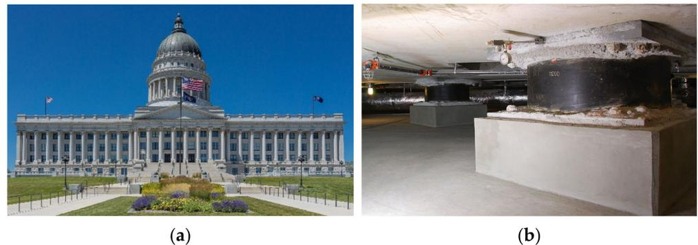
**Figure 3.** Utah State Capitol building (a) and the seismic dampening widgets (base isolators, (b)).
