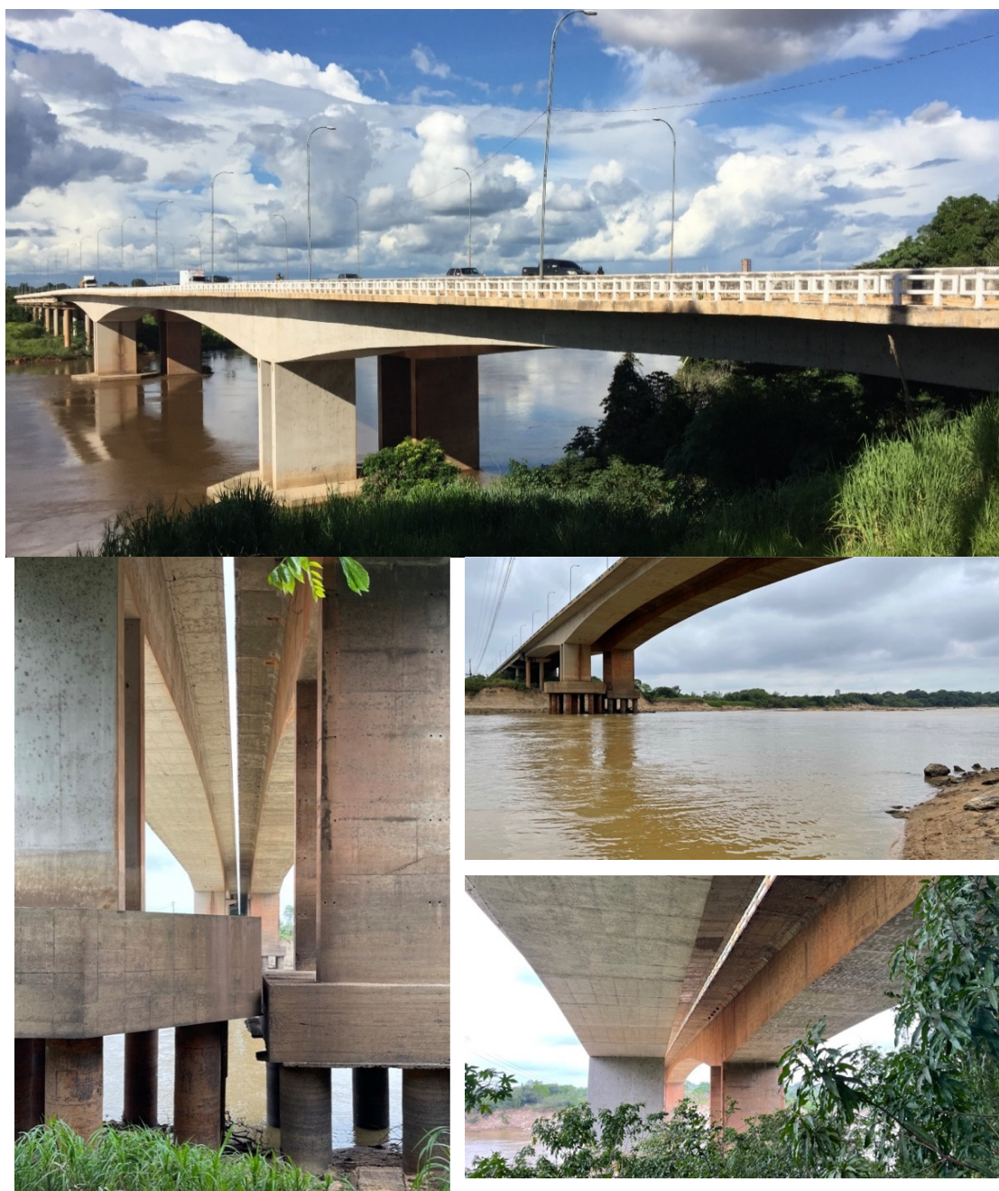
Figure 15. New (left) and old (right) bridges over the Itacaiúnas River.
