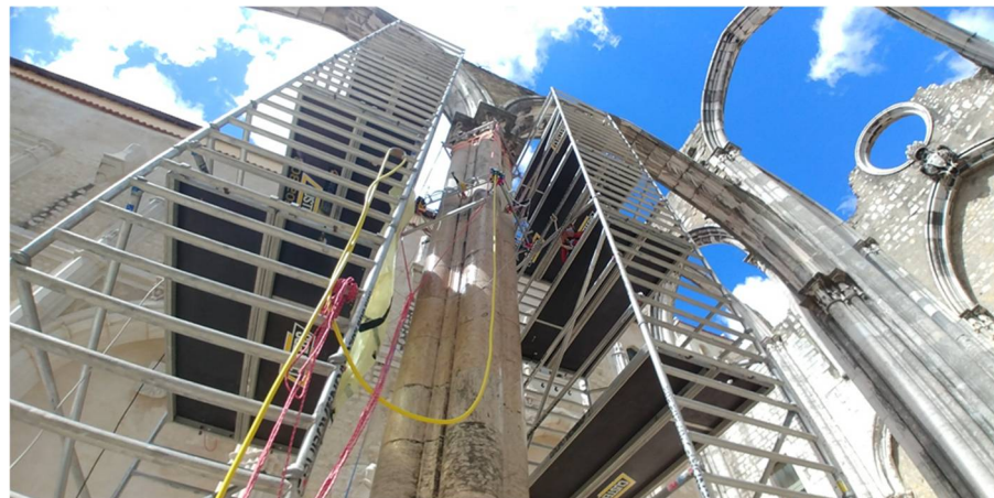
Figure 20. Tomography system inspecting the shaft.
