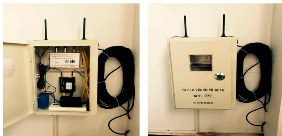
Figure 13. The installation of the seismic sensor in a village hall in Sichuan.
