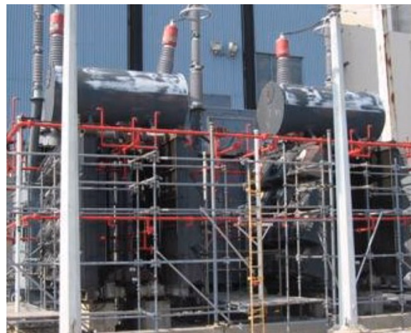
Figure 4. Site operating GE 980MVA Step-Up transformer.
