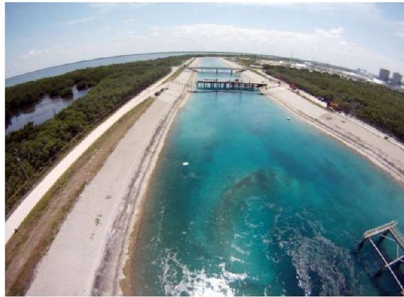
**Figure 2.** The study site: the entrainment canal at St. Lucie nuclear power plant facility located on south Hutchinson Island, Florida. Permanent mesh barriers are located underneath each bridge, keeping marine fauna in the entrainment at the forefront of the photograph. Photo credit: Serge Aucoin.
