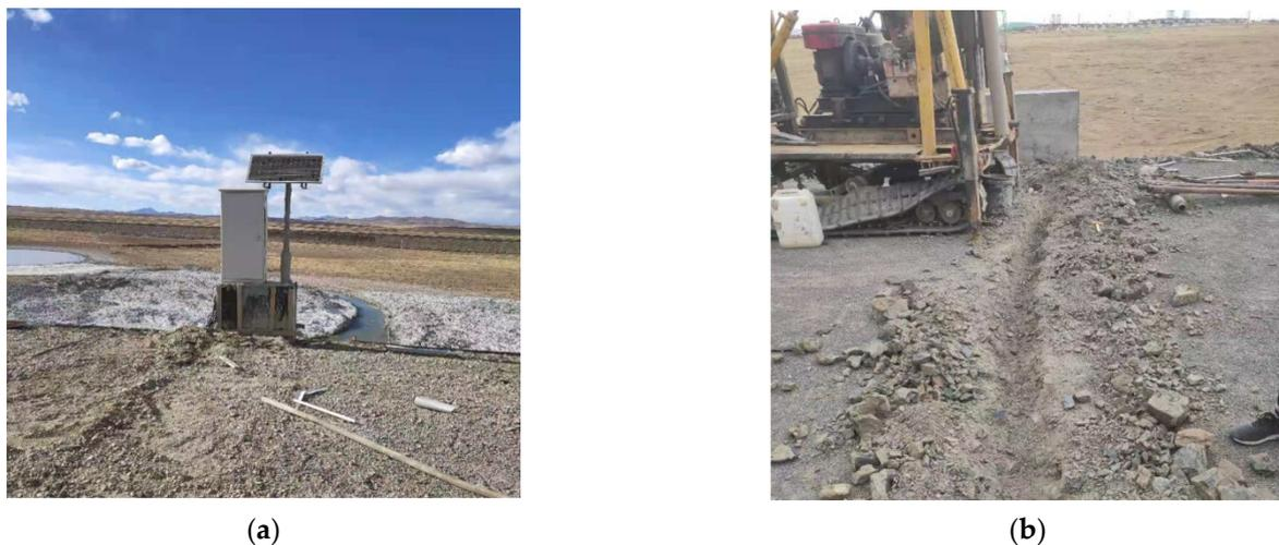
**Figure 5.** Field installation diagram of the instrument at section K3604 + 300. (a) Monitoring box and solar power supply module of section K3604 + 300; (b) wiring groove construction.
