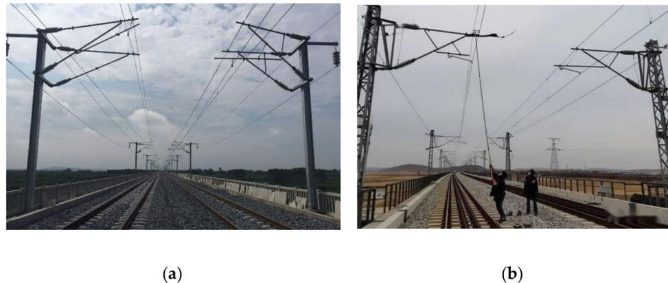
**Figure 1.** The struct of OCS and manual monitoring method: (a) overhead contact system; (b) manual monitoring method.
