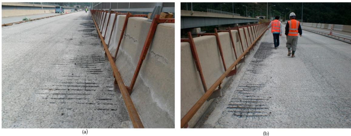
**Figure 13.** Actual concrete condition after removing the asphalt overlay and deteriorated concrete using a high-pressure water-jet machine in the target bridge (“J” bridge) after the GPR survey: (a) area 1 and (b) area 2 (see Figure 11).
