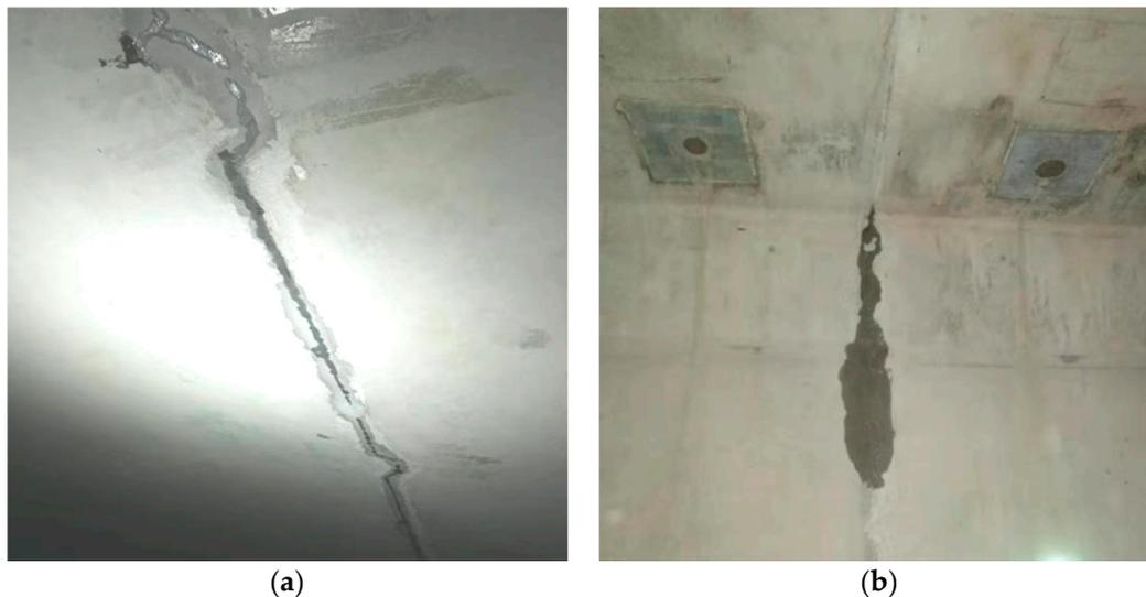
**Figure 1.** Leakage in the box girder of a newly constructed precast segmental bridge. (a) Leakage in the top flange; (b) Leakage in the web.
