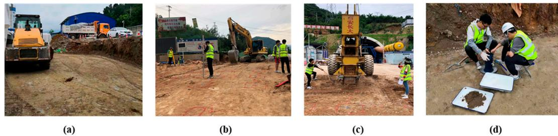
**Figure 15.** Subgrade construction of bid section-06 of Huangling-Yan'an Expressway: (a) layered filling; (b) laying up tamping point; (c) reinforcing subgrade; (d) measuring compactness.
