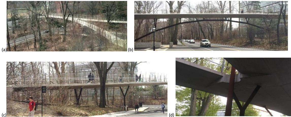
**Figure 1.** Streicker Bridge: (a) near-plan view: main span and approach legs, (b) main span: deck stiffened arch, (c) monitored SE leg: curved continuous girder, and (d) springing of main span.
