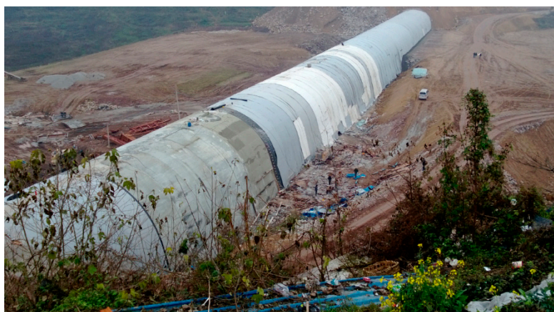
Figure 5. Open-cut tunnel in the backfill process.
