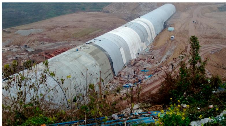
**Figure 5.** Open-cut tunnel in the backfill process.
