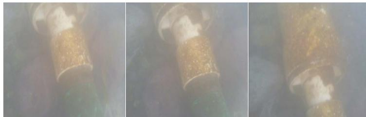
**Figure 22.** Underwater images of current status of connections between PVC pipes.
