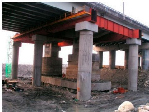
Figure 1. Temporary support steel frame.
