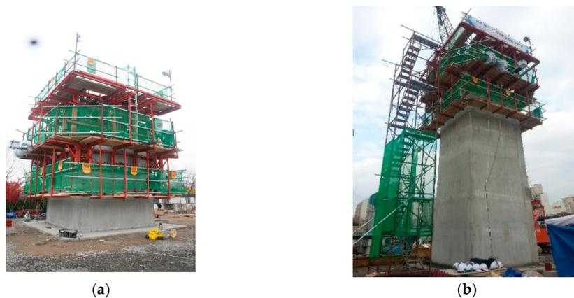
**Figure 13.** Construction of the single concrete tower: (a) during construction and (b) at completion.
