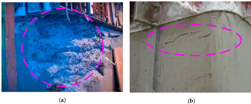
**Figure 1.** Results of improper form lifting: (a) premature form removal and (b) delayed form removal [5].
