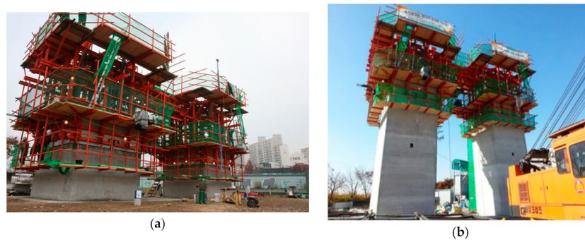
**Figure 18.** Construction of the twin concrete tower: (a) during construction and (b) at completion.
