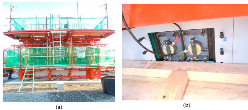
**Figure 10.** Slip-form system for the single concrete tower: (a) the assembled slip-form system and (b) the ultrasonic module installed at the bottom of a Glass Fiber Reinforced Polymer (GFRP) panel.
