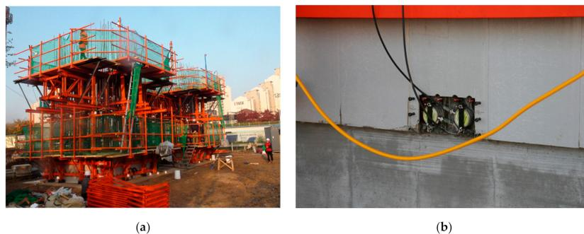
**Figure 15.** Slip-form system for twin-shaft concrete tower: (a) assembled slip-form system and (b) ultrasonic module installed at the bottom of a GFRP panel.
