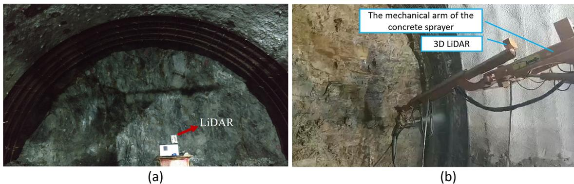
**Figure 4.** The LiDAR in the real tunnel. (a) Data collection site; (b) practical application.
