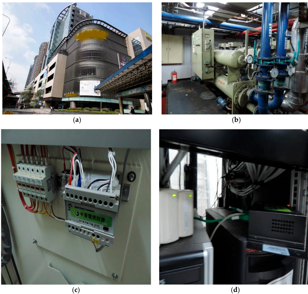
Figure 1. A real test site for presenting artificial intelligence (AI)-assisted heating ventilation and air conditioning (HVAC) control performances. (a) The case study facility; (b) the chiller system including 6 chillers installed in the building; (c) a power meter for measuring the energy consumption; (d) a networked temperature/humidity sensor module for detecting the necessary parameters for the HVAC control.
