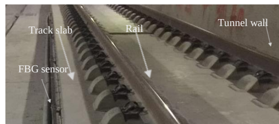
Figure 1. High-speed rail (HSR) slab track system in the tunnel.
