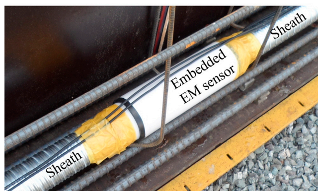
Figure 3. Installation of an embedded EM sensor.
