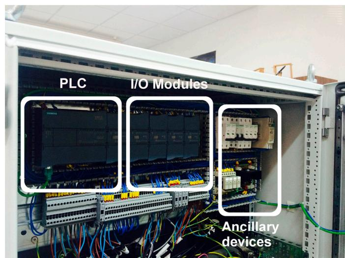
Figure 9. Automation subsystem.
