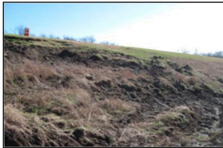
**Figure 1.** Slough or slump slide on a levee.
