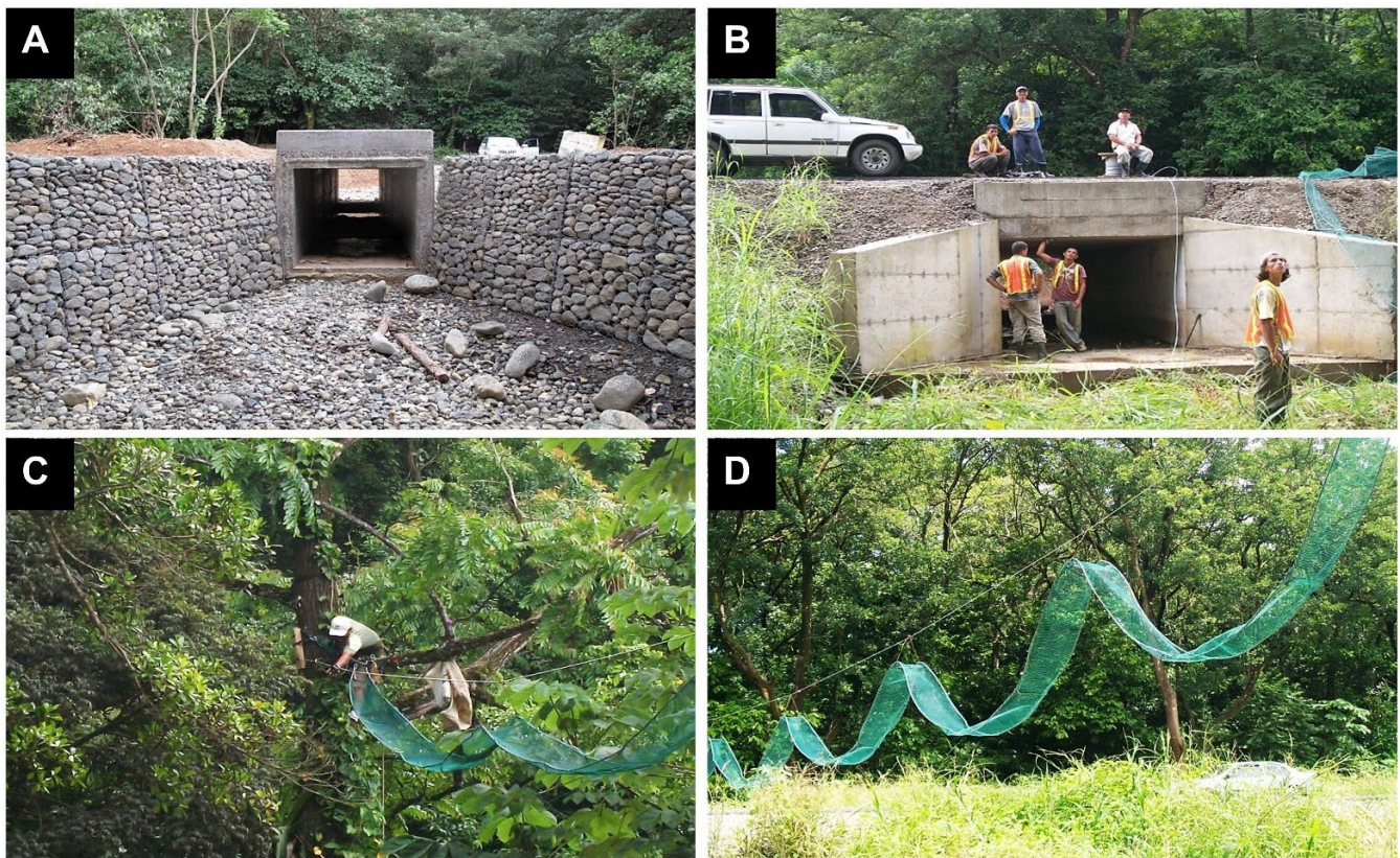
Figure 3. Construction of the wildlife-crossing structures at Hacienda Barú National Wildlife Refuge, circa 2010: (A,B) tunnels under construction and (C,D) bridges under construction. Source: Hacienda Barú National Wildlife Refuge.
