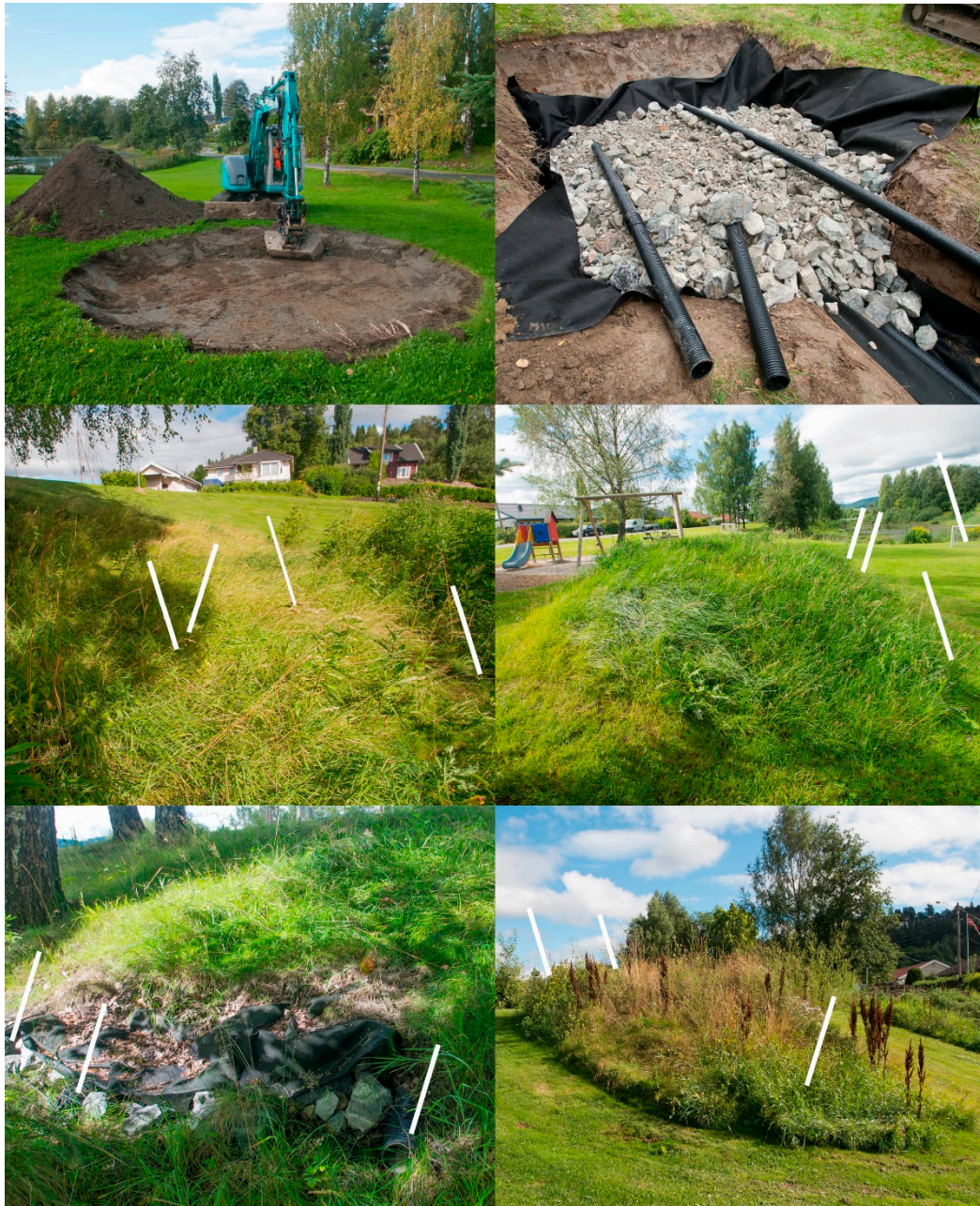
Figure A2. Photos of excavator at work during construction of Hotel 2 ( top left ), drainage pipes, geotextiles and rocks of Hotel 1 ( top right ), and final result of Hotel 1 ( mid left ), Hotel 2 ( mid right ), Hotel 3 ( bottom left ) and Hotel 4 ( bottom right ).
