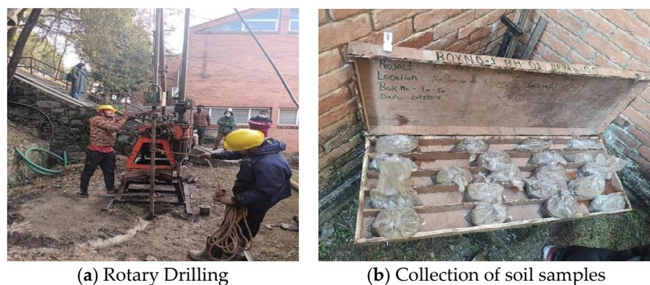
**Figure 4.** Soil investigation works by drilling method. (a) Rotary drilling, (b) collection of soil samples.
