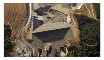
Figure 7. Upstream embankment construction.
