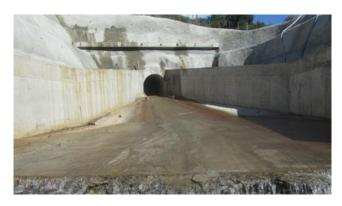
Figure 3. Diversion tunnel exit portal.
