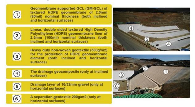
Figure 5. Description and installation of the composite lining system.
