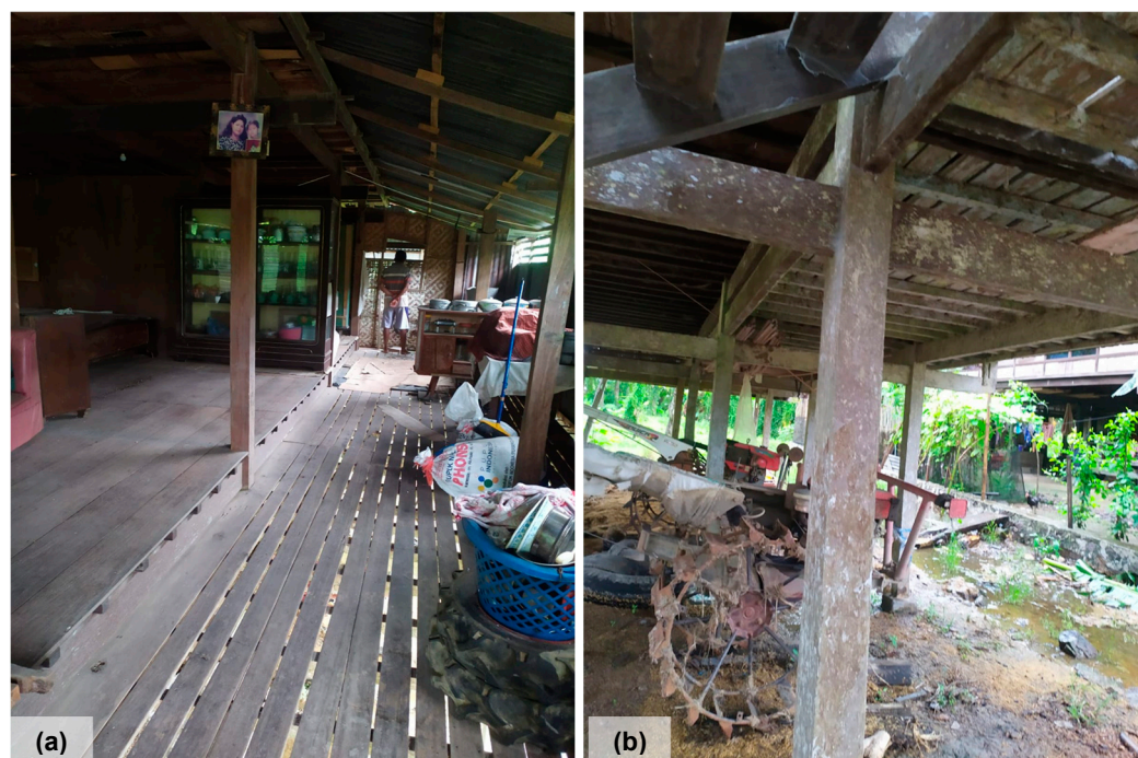
Figure 3. “Tamping” circulation spaces in Bugis–Makassar traditional houses to act as evacuation routes during natural disasters, including earthquakes. A view from inside the house (a) and a view from outside the house (b).
