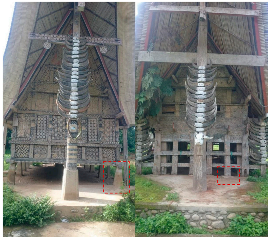
Figure 2. Mountain stone foundations support the pillars of Tongkonan houses.
