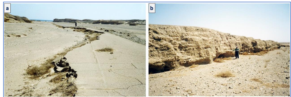
Figure 14. Selective examples of flood validation through field observation (a) damage to the road at the outlet of the Wadi Umm Gheig. (b) Flood impact on the undercutting of 4 m terraces in the Wadi Umm Gheig.
