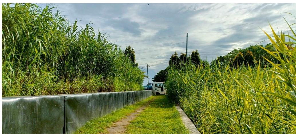
**Figure 1.** Vertical flow (left side) and horizontal flow (right side) constructed wetlands in the City of Bayawan. Photo taken by the authors.
