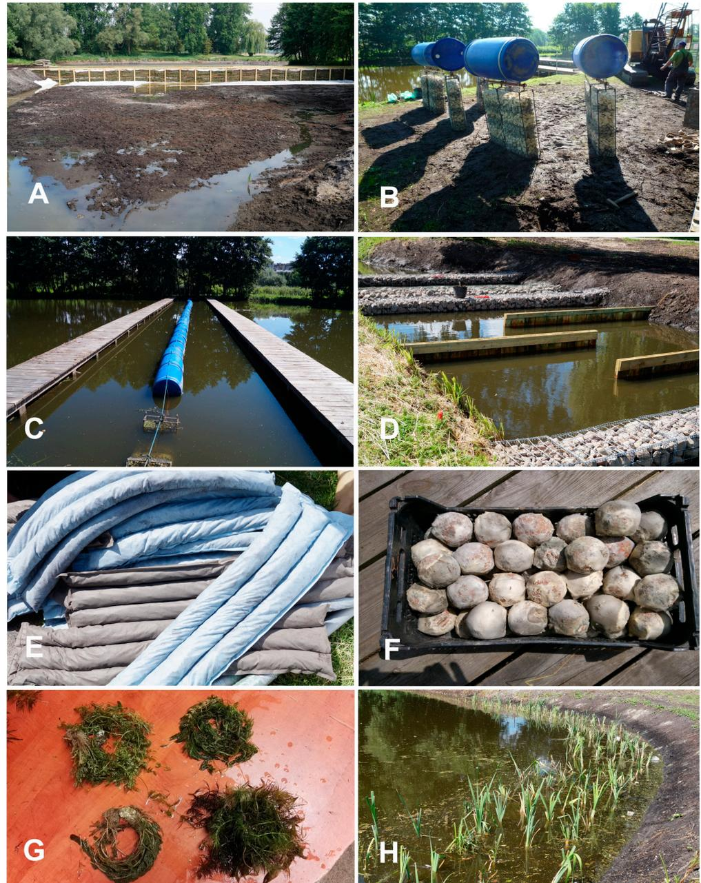
**Figure 4.** Structural and biotic elements of the SED-BIO system: (A)—a wicker gabion on a drained pond (section A); (B)—floats with a mineral filter, (C)—two wicker gabions with a mineral filter between them (section A); (D)—view of section B; (E)—specially prepared mattresses with denitrification deposit; (F)—Micro-Dictum preparation; (G)—wreaths of submerged plants specially prepared for planting; (H)—planted *Typha* and *Glyceria* in the littoral zone (section A).
