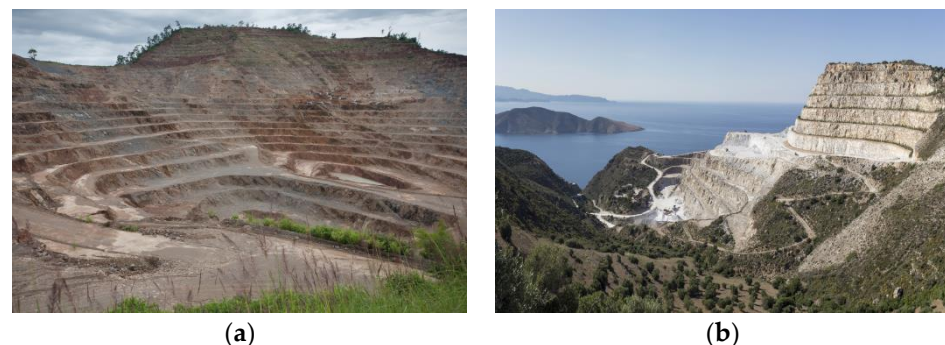
Figure 1. Examples of berms installed on actual slopes: (a) Slopes with berms in Thailand (Roengrit Kongmuang/Shutterstock.com; accessed on 9 March 2021); (b) slopes with berms in Crete, Greece (Gestiafoto/Shutterstock.com; accessed on 9 March 2021).
